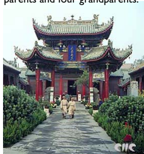
The Assembly Hall of Shanxi, Shaanxi and Gansu, Henan Province
