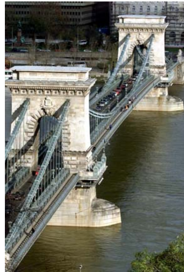
Above, The Chain Bridge over the Danube. EPA PHOTO / ATTILA KISBENEDEK
